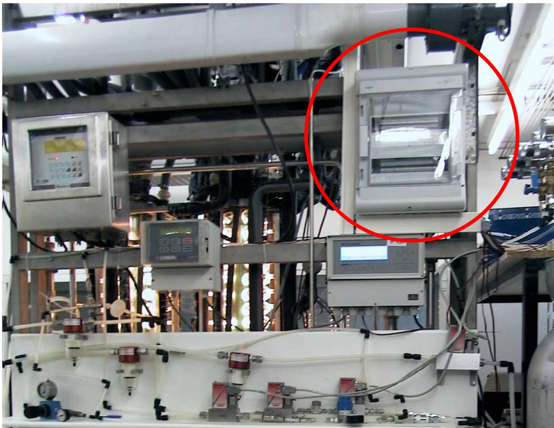
**Figure 3: Close view of the location of the auxiliary connection panel (inside red circle) on the backplane of the compartment IVa bioreactor.**
