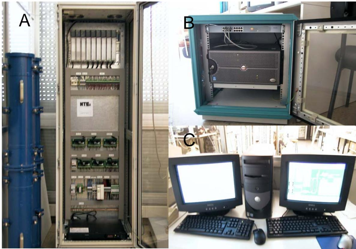
**Figure 2: Close up views of compartment IVa control system. A: Controller’s rack. B: Master controller and database server computer, with a 3Com Ethernet Switch. C: perspective of the user interface Dell computers.**
